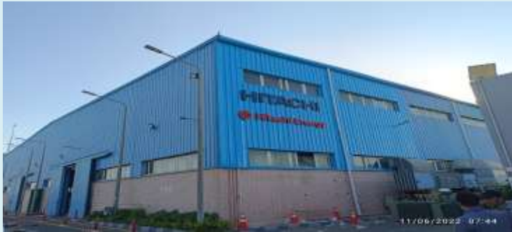
HITACHI TRANSFORMERS FACTORY, 10TH OF RAMADAN. EGYPT
